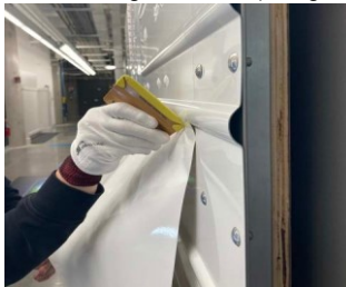
Figure 4. Squeegee the bottom of the corrugation.
