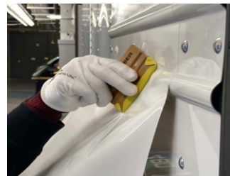
Figure 3. Squeegee the crown of the corrugation.
