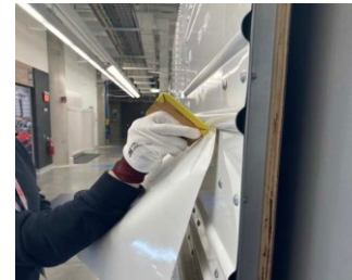
Figure 5. Bead the lower valley.
